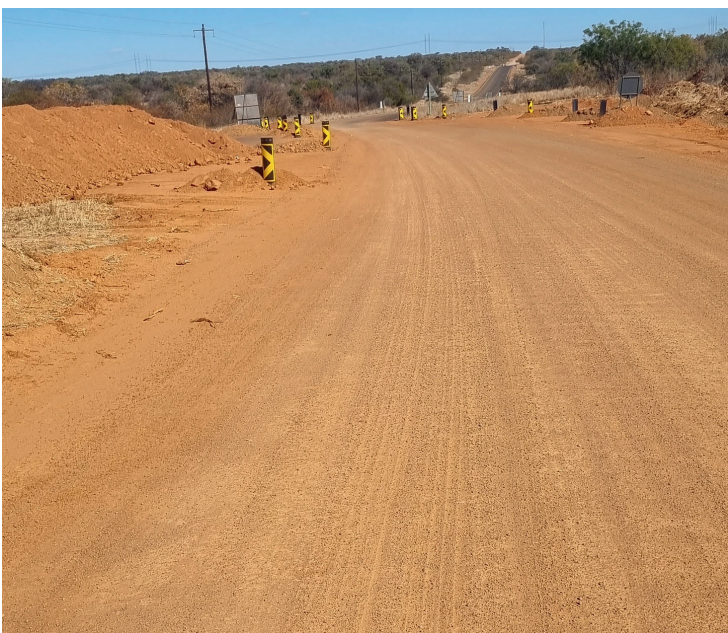
Photo: Road work
